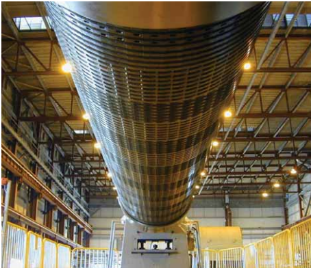
Middle East: Balancing generator rotor in power station upper floor.
